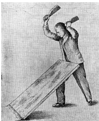
DRAWING OF POPOV'S SOUND DEVICE THAT IMITATES GUN SHOTS. EARLY 1940s.
